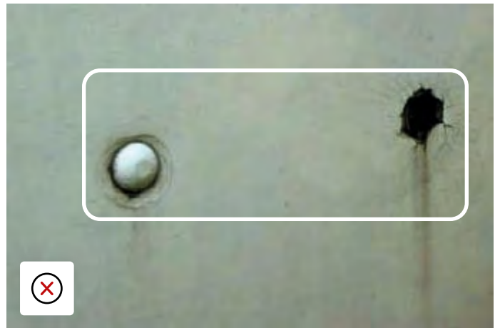
Bolts through GRP side panels.
