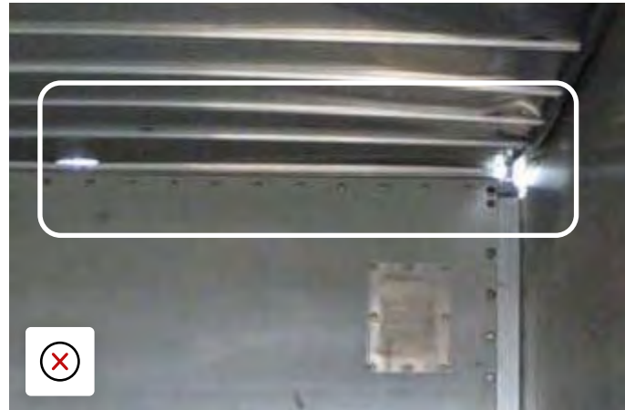
Damage to front roof sheet
